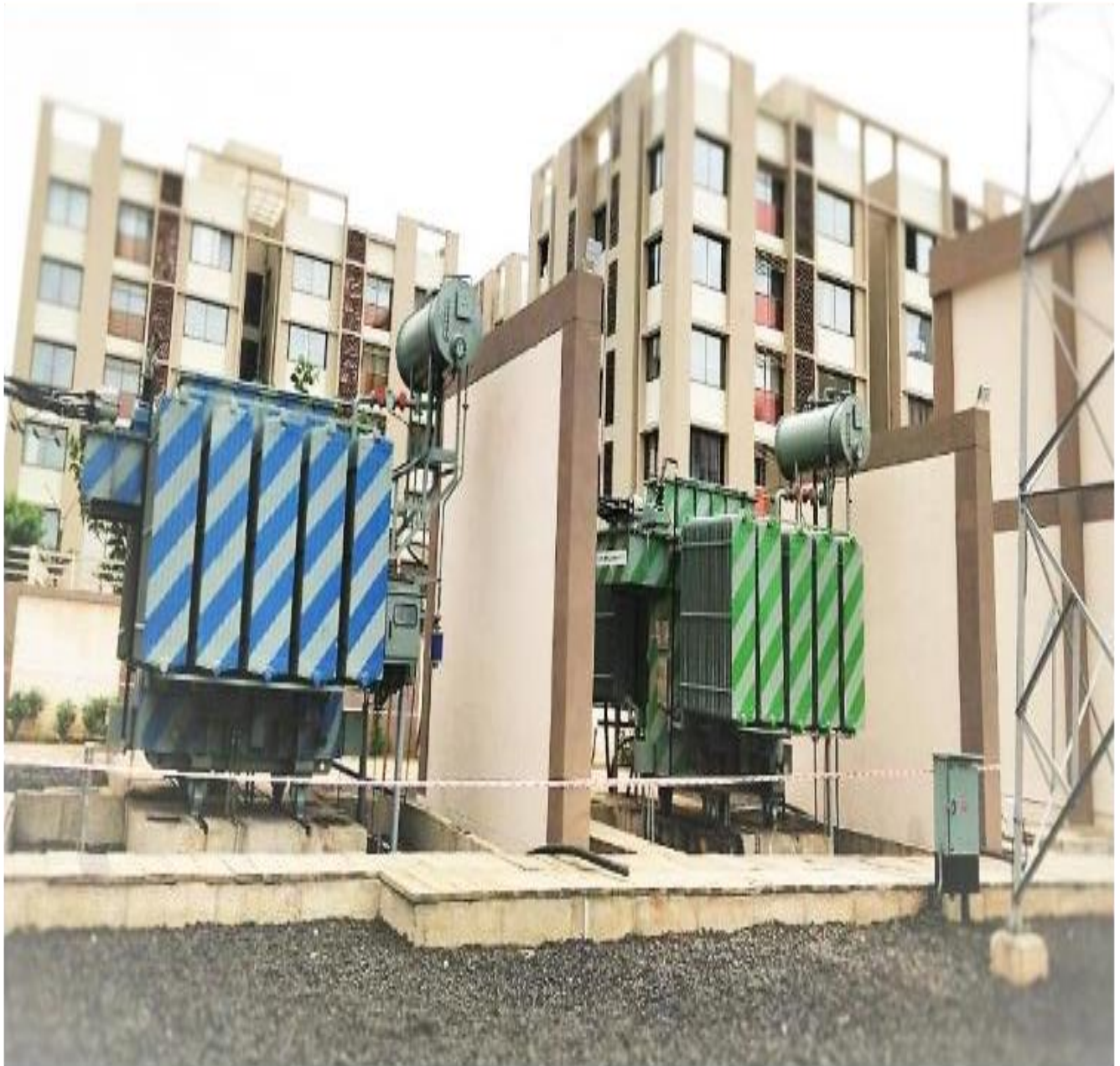
Actual site image of Atlanta make Natural Ester oil filled transformer
